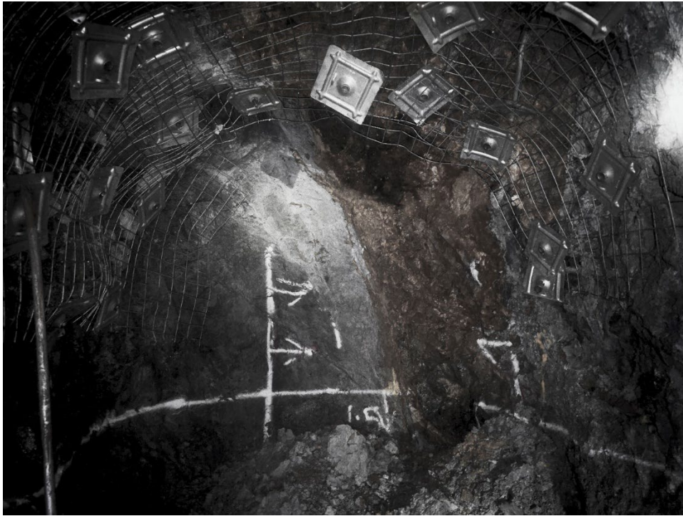
Figure 4. Photograph of Tolukuma 1560 Ore Drive, Cross Cut 2, facing north, exposing the extensive mineralised epithermal quartz vein breccia.
