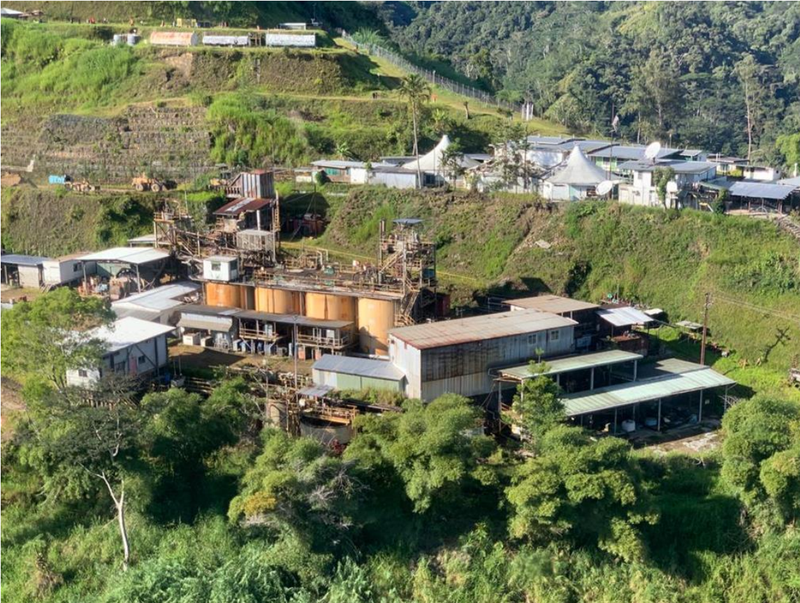
Infrastructure in place
