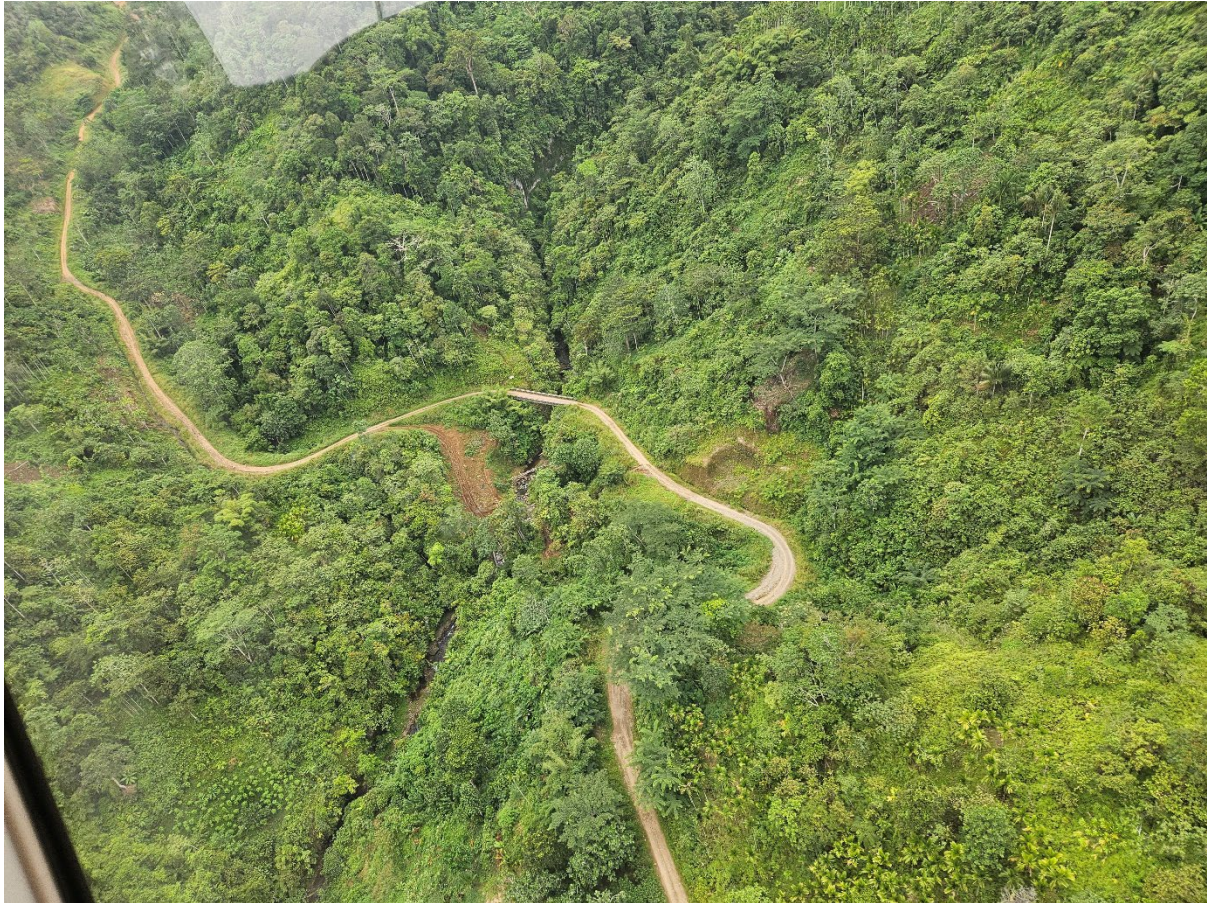
Figure 5: New Tolumuma Access Road
