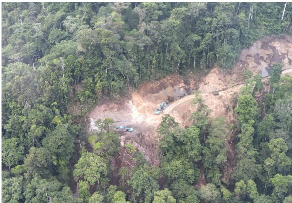
Figure 27 - Tolukuma site access road currently being constructed.
