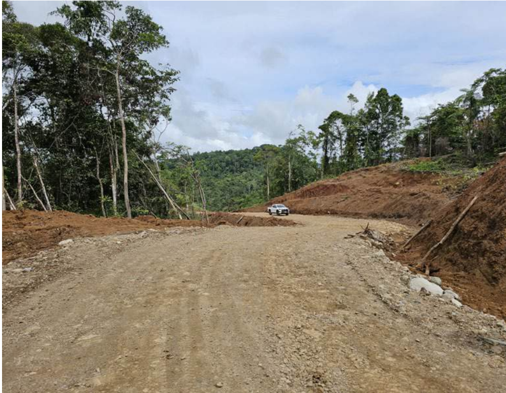
Photo 1: Section of the New Tolukuma Access Road
